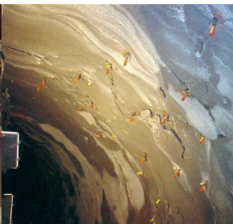
Figur 12, GFRP bultar i Vernia tunnel
