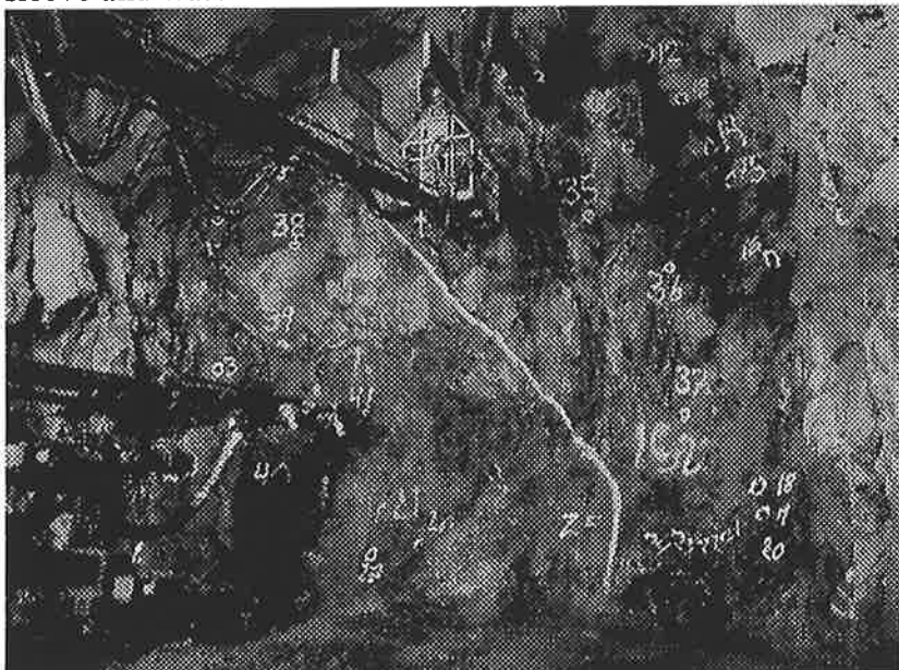
Figure 2 Drilling of observation holes. The fan consists of 32 grout holes in the periphery and 10 observation holes in the middle. The separator between equal Lugeon sums is shown.
